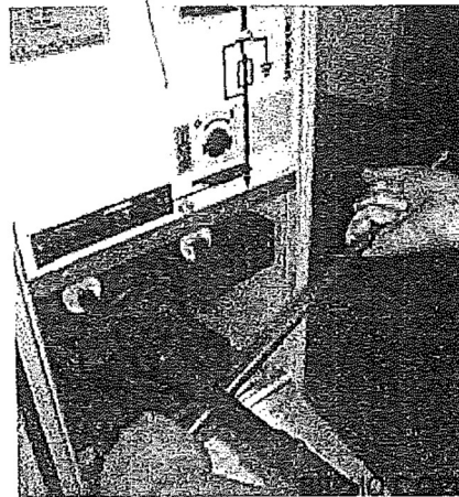
5. Applying the operating handle and turning anti-clockwise opens the fuse canisters.
